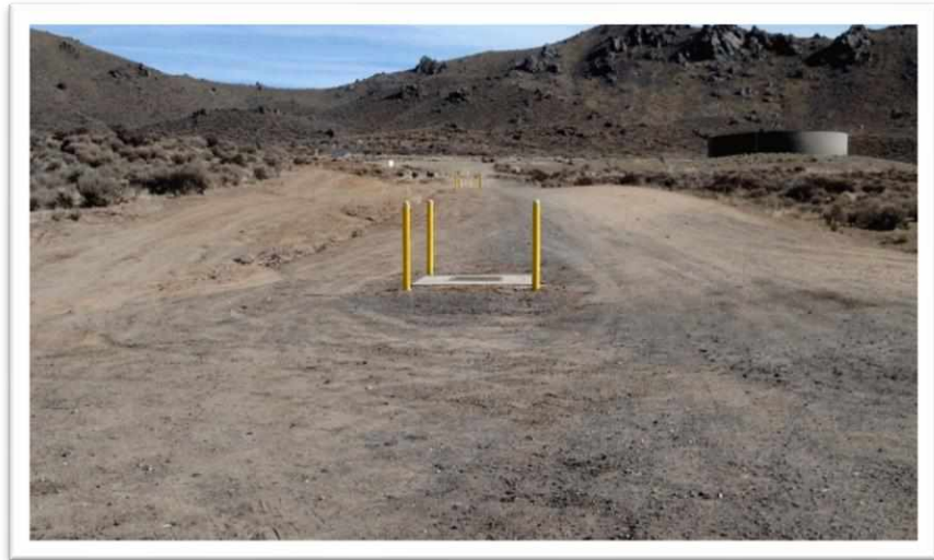
Photo 7. Koontz Lane below the water tank
